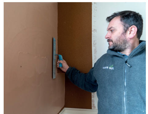
Plaster skim directly over the SprayCork
